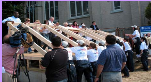
"Raising the wall" during Habitat for Humanity
